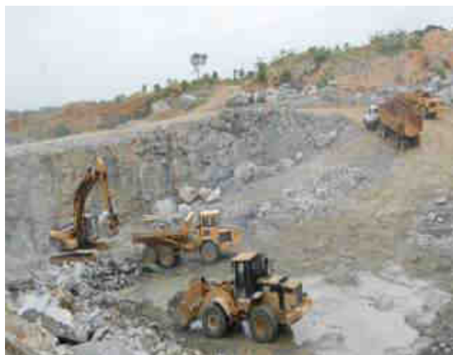
Figure 1 Ashaka Cement Quarry Site
